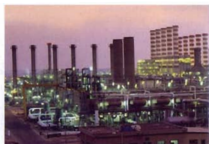
Figure 5 The Ras Abu Fontas combined power and desalination plant, near Doha, Qatar. The whole plant generates over 1600 MW of power using several gas turbines and produces about 100 ML per day of fresh water from sea water using the waste heat from the gas turbines.
