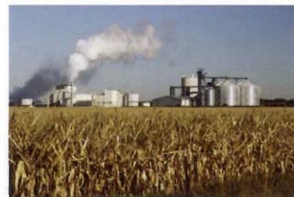
Figure 1 A biofuel production plant
