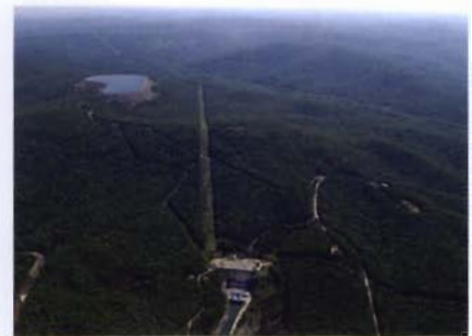
Figure 5 Taim Sauk pumped storage plant
