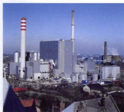
Figure 4 The Elcho combined heat and power plant in Poland, which is capable of supplying 226 MW of electricity and up to 500 MW of district heat
